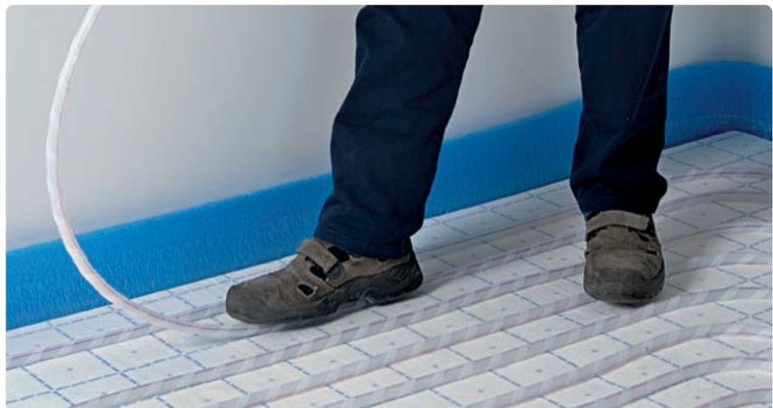
Reposition the pipe and secure in place by simply treading on it again. You can also lift and refix using your hands
